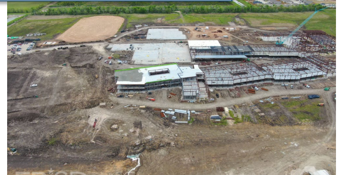
HS 12 Construction Site
